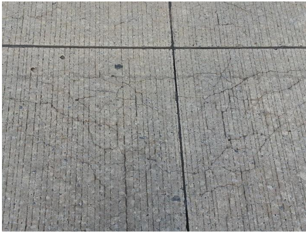
Fig. 1.1-2 –Typical deterioration in concrete pavements due to F/T and ASR (by Richard Deschenes Jr.).
