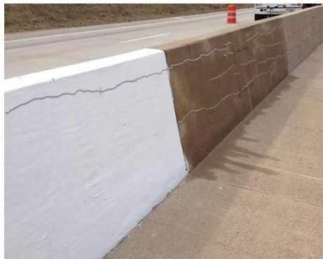
Fig. 3.3-2 –Barrier sections treated with elastomeric paint (left) and silane (right) (by Richard Deschenes Jr.).
