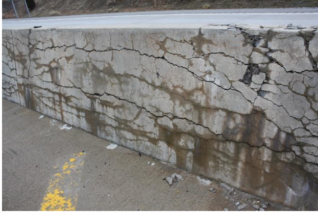
Fig. 1.1-1 –Typical deterioration in concrete barriers due to F/T and ASR (by Richard Deschenes Jr.).
